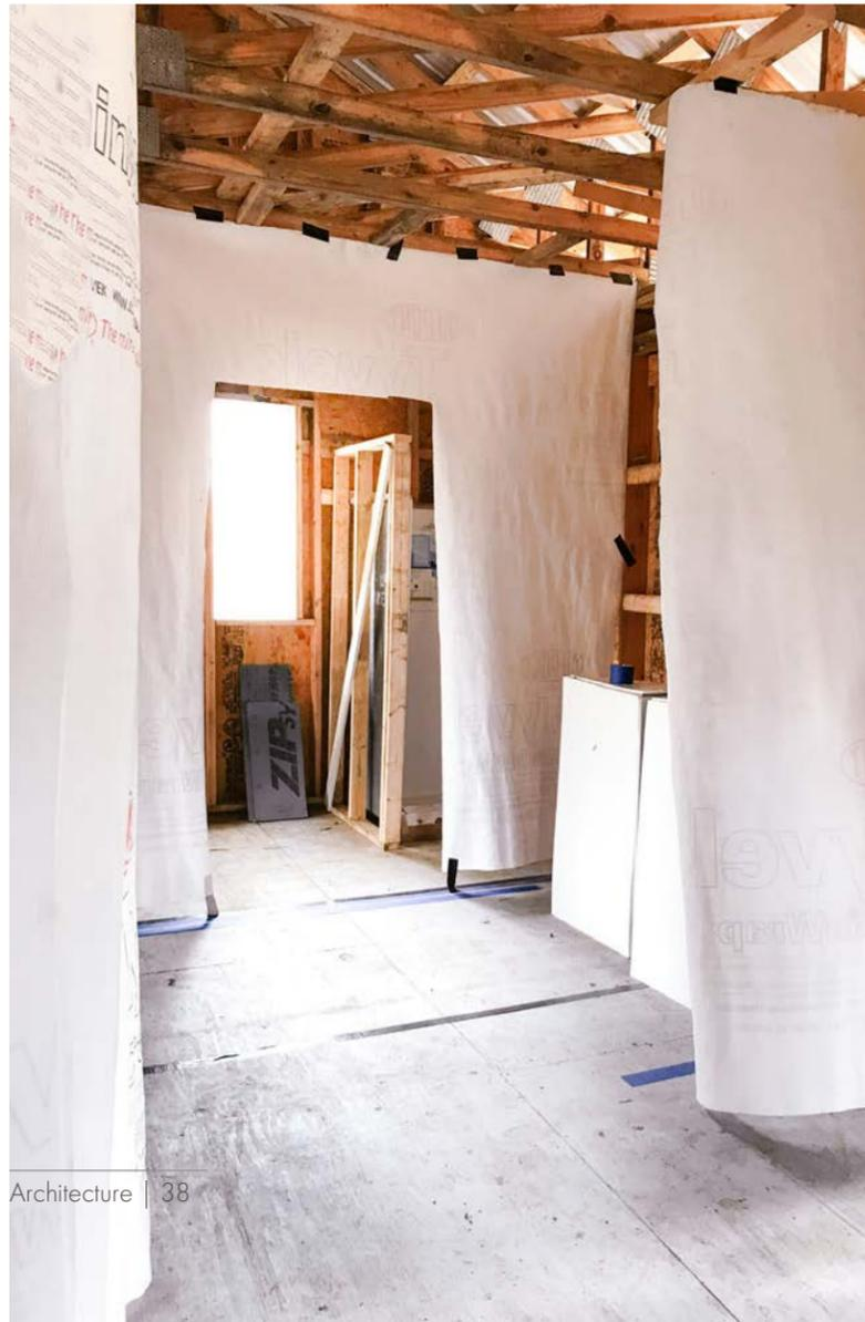
Several modifications were made on site. For example, a casing was built over the nook to provide a more formal separation of the spaces (right). The nook's fin wall was also extended to provide more storage space and privacy for the utility room. These decisions were made by creating full-scale mockups to analyze the space in full scale (left).
