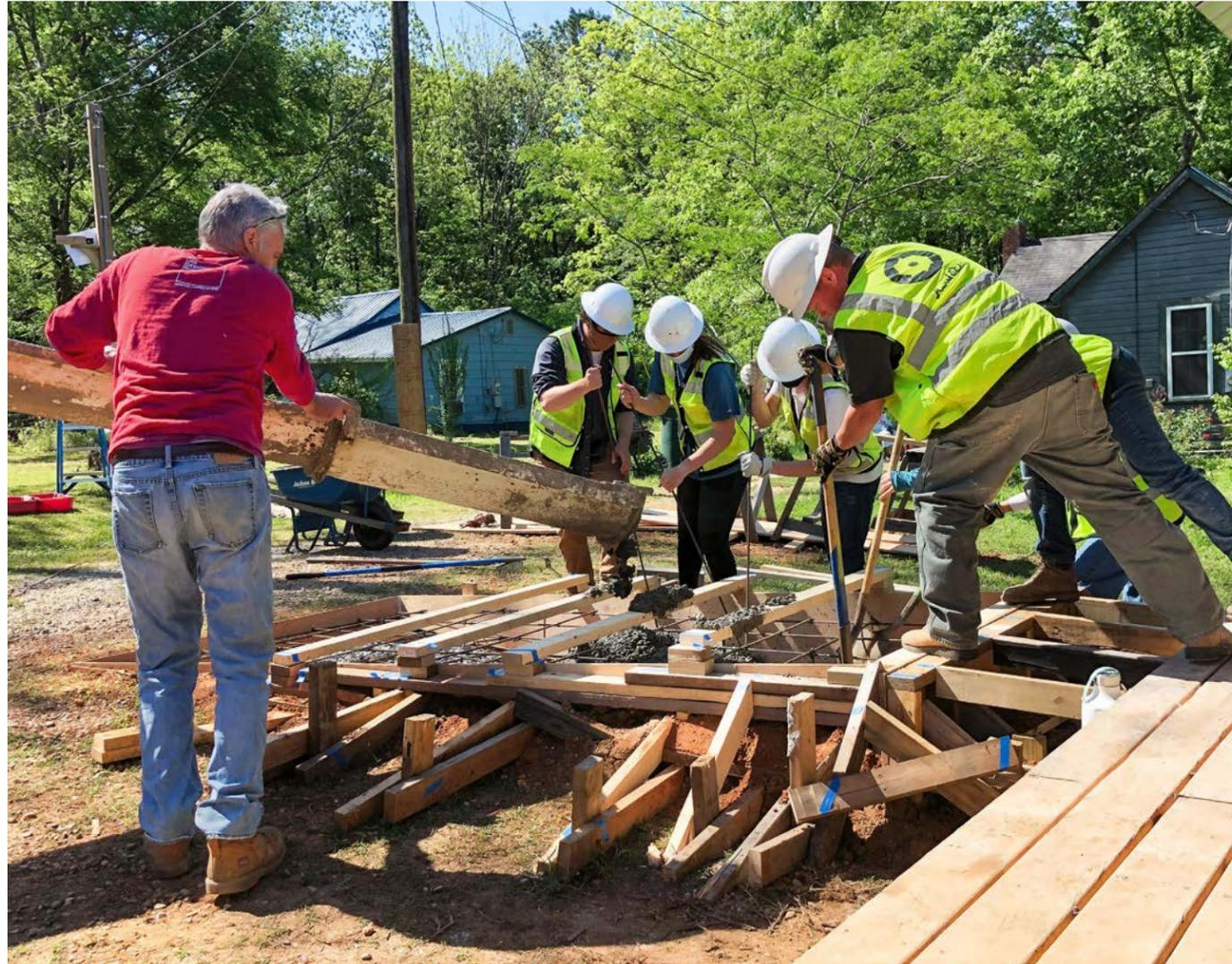
Because our client needed a wheelchair-accessible entrance, we created a 16' concrete ramp with a steel grate for rainwater runoff. Three cubic yards of concrete meant formwork needed to be extremely fortified.
